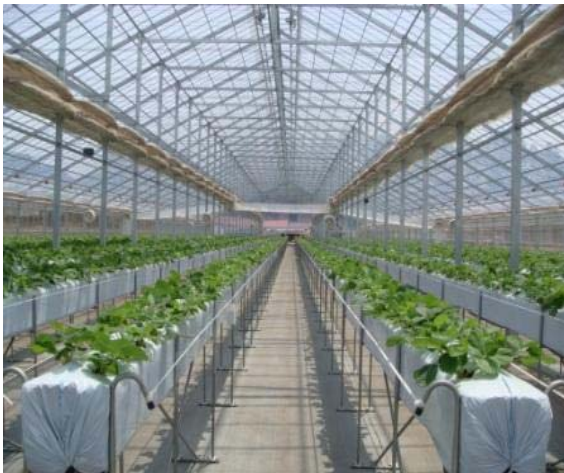
Steel frame greenhouse
